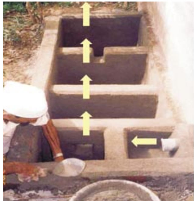
Construction of greywater treatment system
